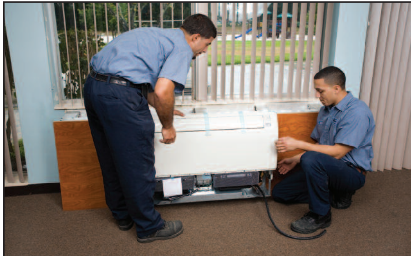
Eugene Roman, Garrison Mechanical technician, and Carlos Roman, tech, complete a Fujitsu air handler installation.
