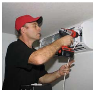
Technician Nelson Vokey installs an air handler.
