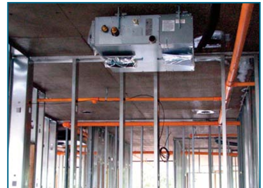
A combination of wall mounts and concealed slim ducts units were used inside the condo complex.
