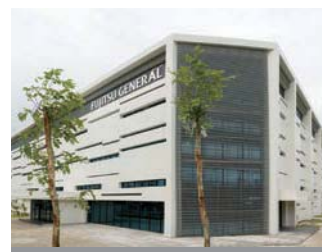
R&D Center in Fujitsu General Engineering (Thailand)
