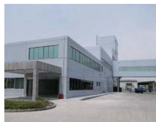
R&D Center in Fujitsu General Engineering (Thailand)
