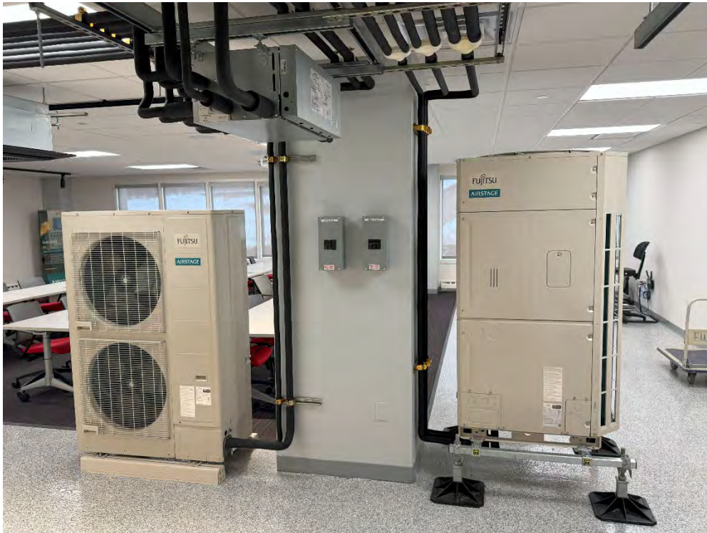
Many of the training opportunities at the new facilities focuses on Fujitsu's AIRSTAGE Commercial and light commercial heat pump products.
