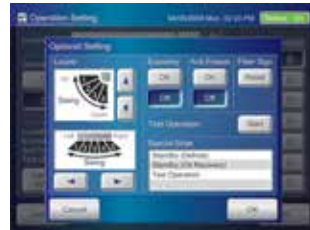
Indoor units operation monitoring
