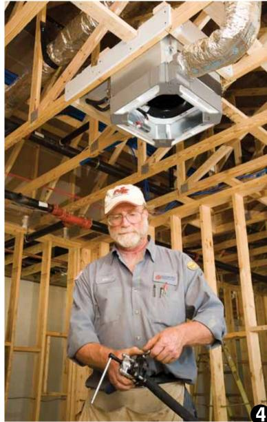
demand, and no more," added Herne. Equipped with 20-kW backup heat and  $\rm CO_2$  sensors, the Modine unit will also run whenever the building's air needs exchanging.
