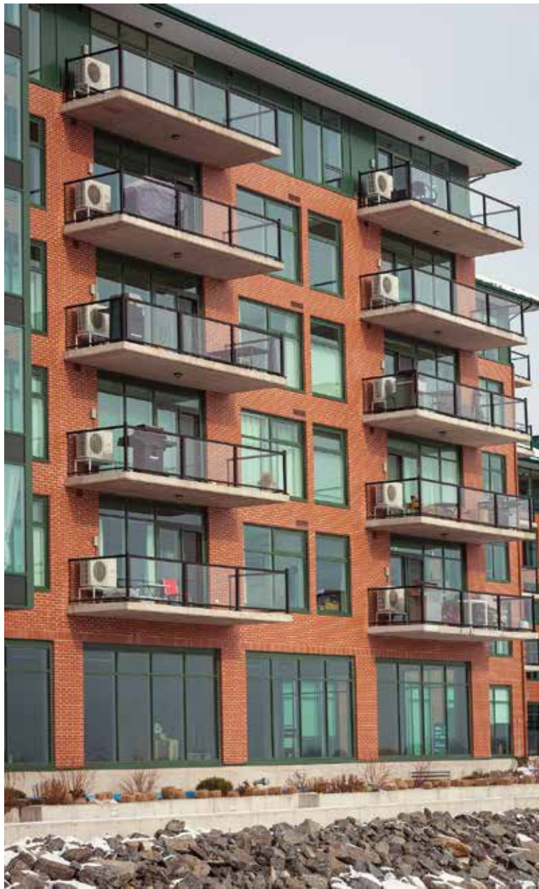
The project includes a total of 79 Fujitsu RLXFZ units for the condo units and one common area.
