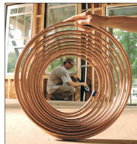
A coil of copper refrigerant line stands ready at the jobsite, where it will transport refrigerant between an outdoor condensing unit and an interior air handler.
