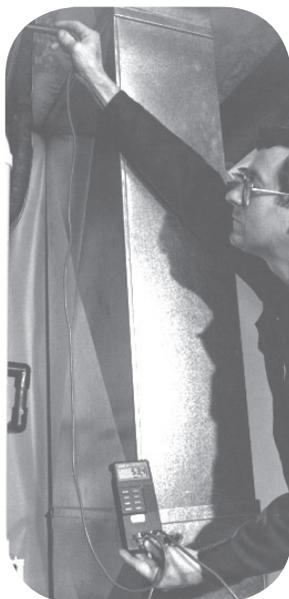
If the measured temperature rise is below the nameplate range, the gas input rate may need to be adjusted or the airflow may be too high. If the gas input is correct, select the next lowest speed tap for the heating function. If the measured temperature rise is above the nameplate range, the gas input rate may need to be adjusted or the duct system may be too restrictive due to undersized ducts. An undersized return duct is a common cause of an overly restrictive duct system.
